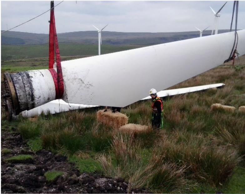
2014 Desmantelamiento de 24 turbinas VESTAS WD34 Coal Clough wind farm in Burnley INGLATERRA (SCOTISH POWER – IBERDROLA)
