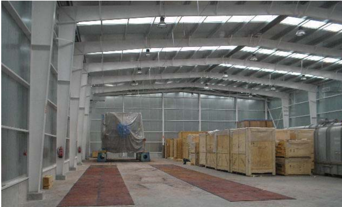
GTG Package Equipment inside the warehouse
