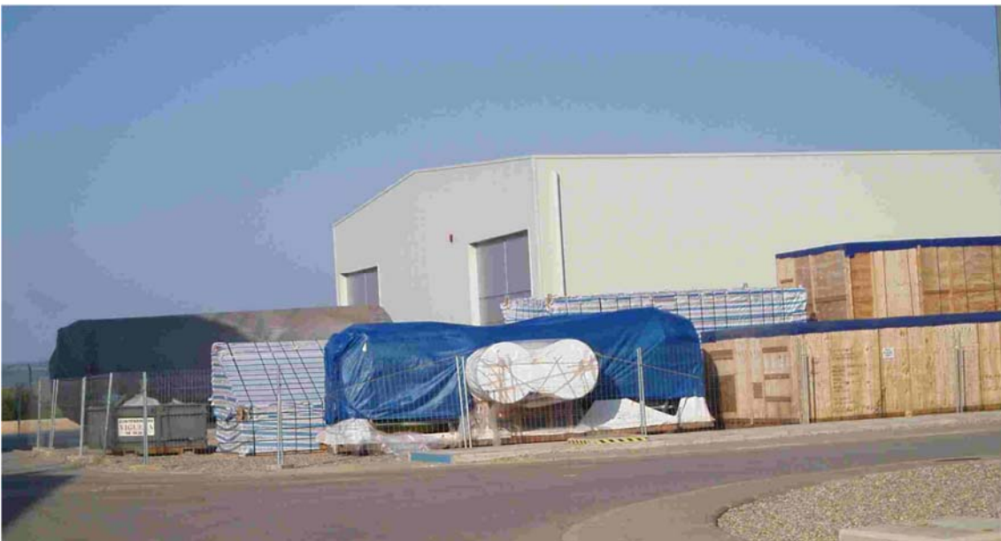
Outdoor storage area for the GTG Package Equipment (1)
