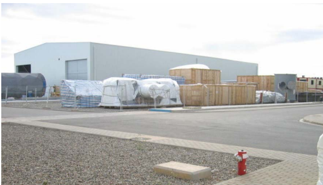
Outdoor storage area for the GTG Package Equipment (3)
